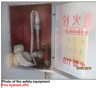
Photo of fire safety equipment Fire hydrant testing (2).JPG
