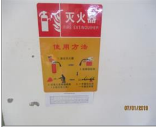
Photo of fire safety equipment Fire extinguisher usage instruction.JPG
